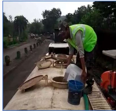
Addition of Liquid Chemical Additive
