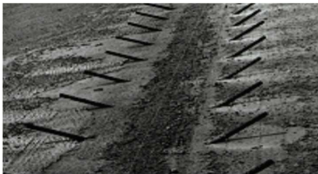
Inserting Bars along longitudinal joint
