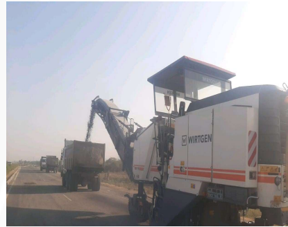
Milling Machine to mill the distressed layer
