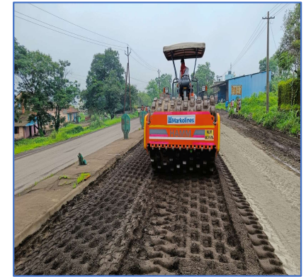
Compaction by Pad Foot Roller
