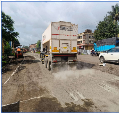
Cement Spreading by Microprocessor Controlled Spreader Truck
