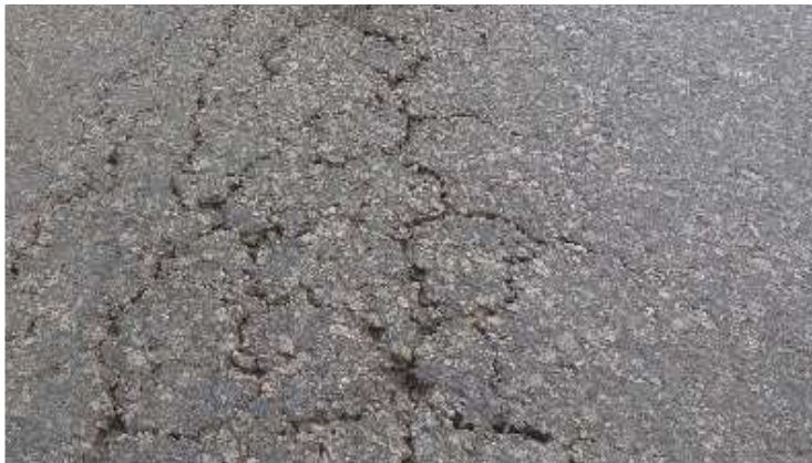
Alligator Cracks
