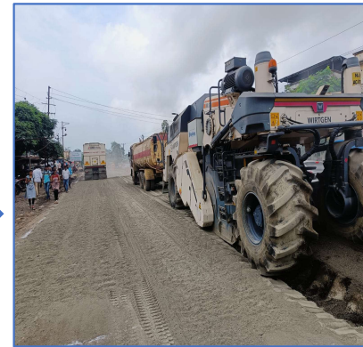
Pulverization of soil with Recycler
