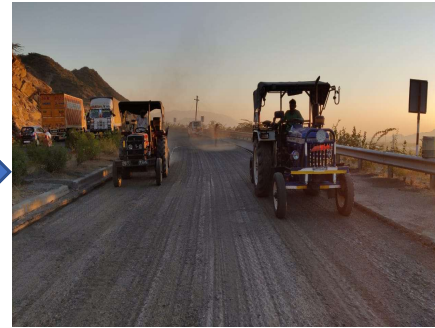
Broomer & Compressor used for cleaning
