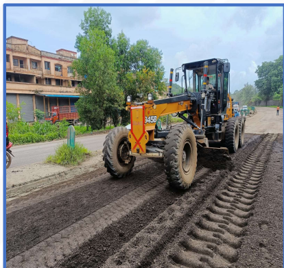
Grading & Profiling with motor Grader
