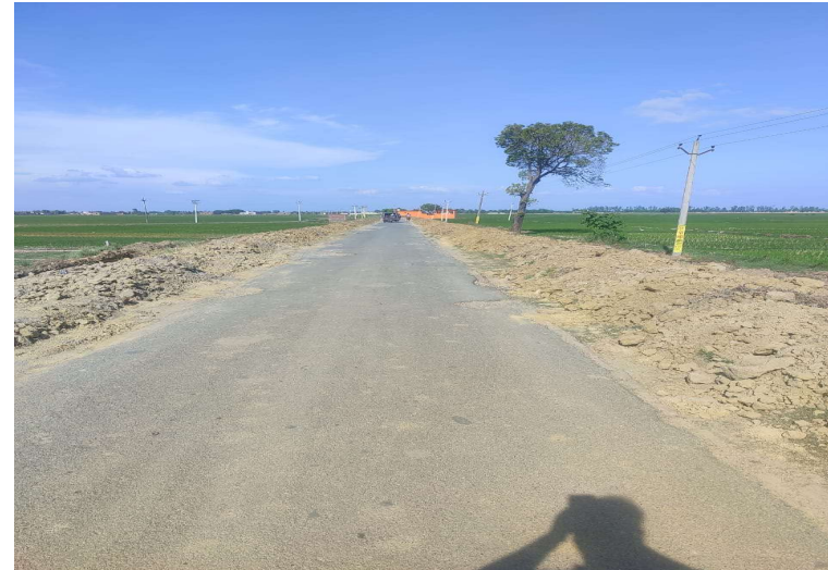
Widening of Existing Road
