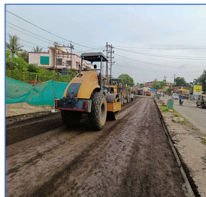
Compaction by Soil Compactor
