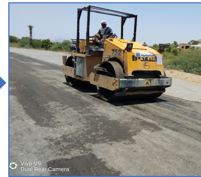
Tandem roller for sealing top layer
