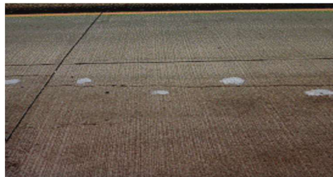
Cross Stitching Along Longitudinal Joint
