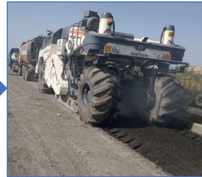
Milling & pulverisation by WR240 Wirtgen Recycler
