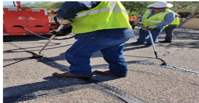
Application of hot sealant
